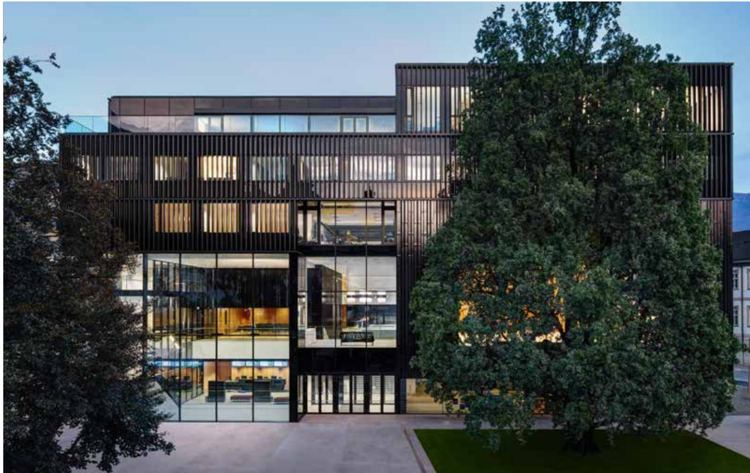
cero III Das Brahms Innsbruck, AT Architect: Erich Strolz, Dietrich Untertrifaller Photos: Dr. Günther Egger Ref. 1647*
