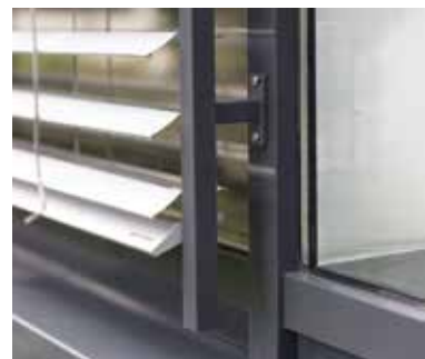
Guiding rail with spacer
