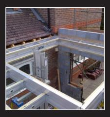
Made from a series of numbered, pre-fabricated sections for ease of installation
